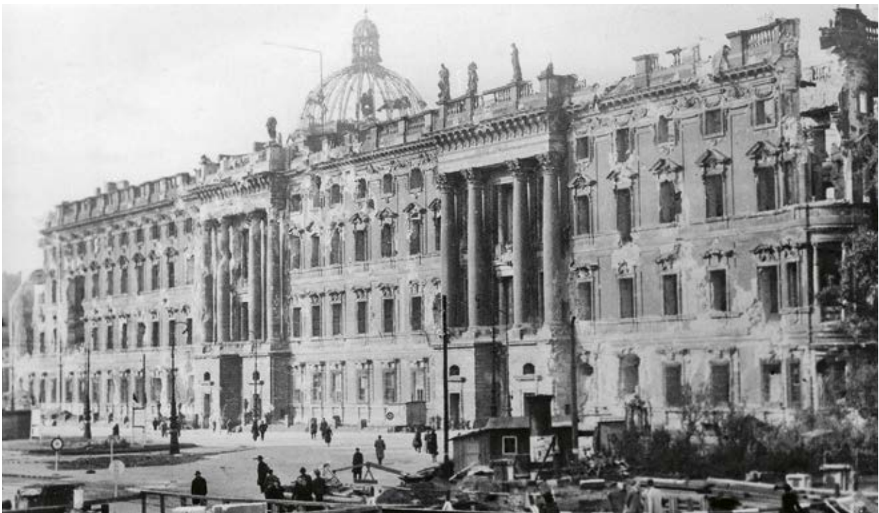
The Palace before the blasting.
