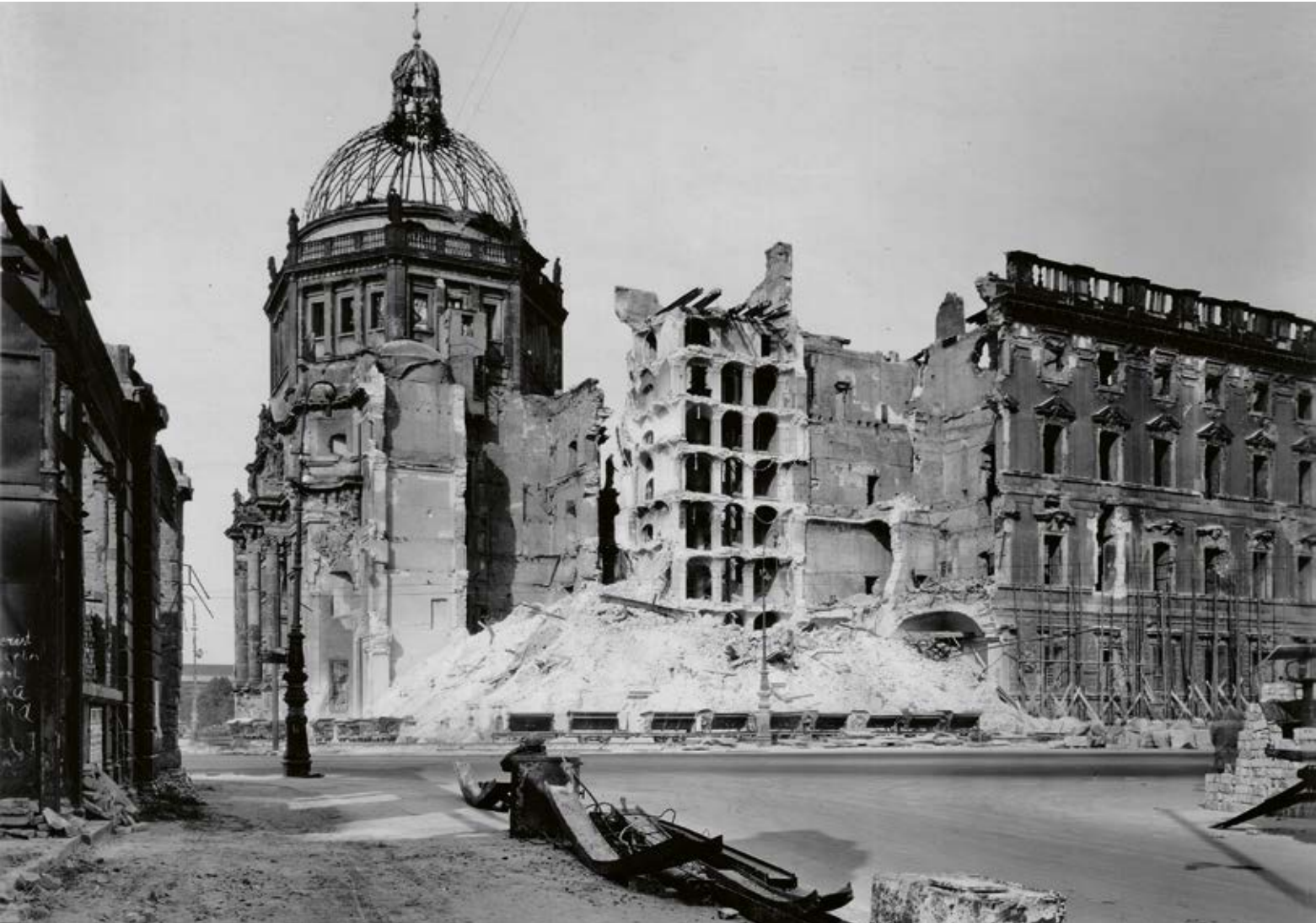
The same motif in 1950: The blasting works have begun. In front of the destroyed façade is a tipping wagon used to dispose of the rubble.
