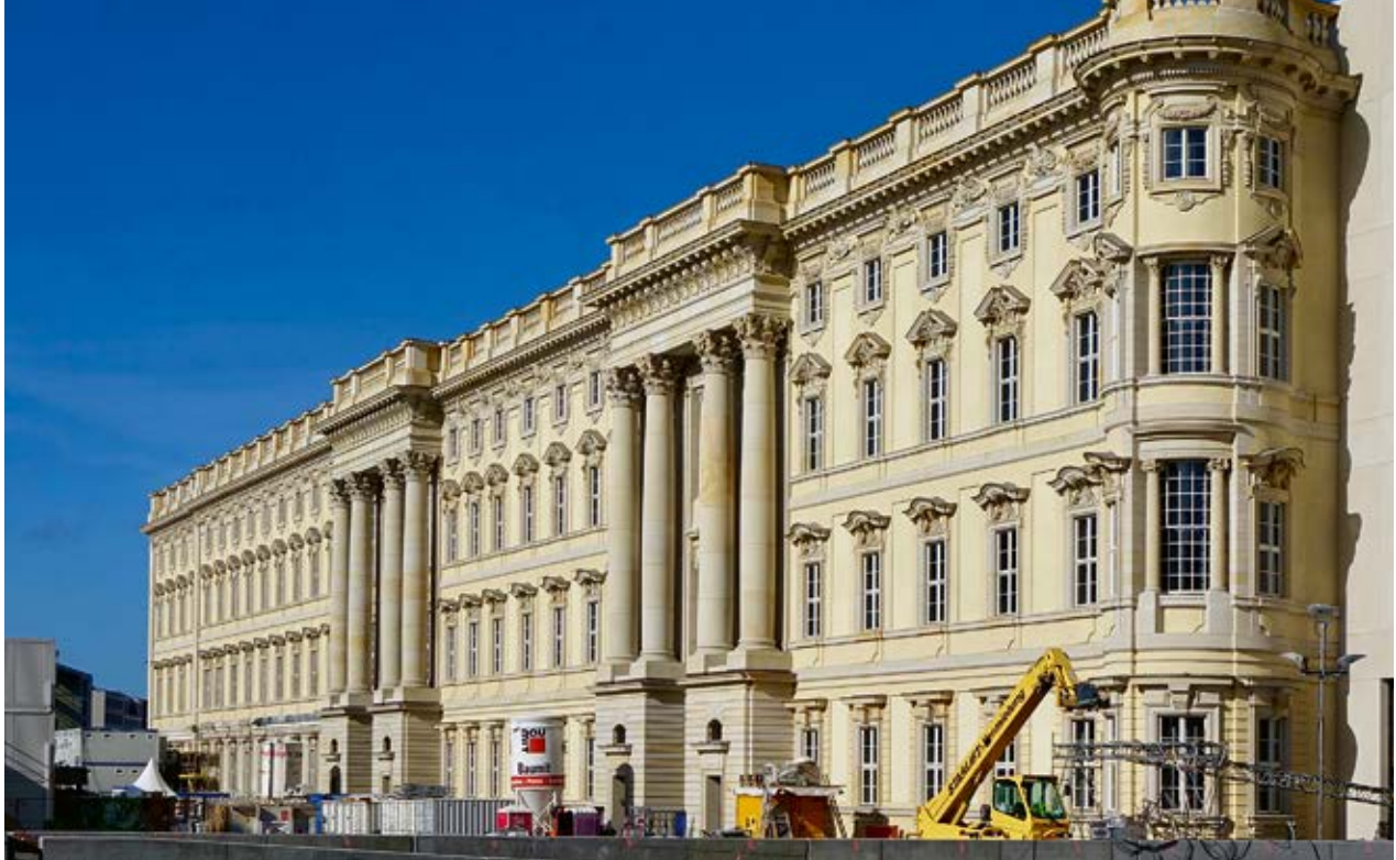
2020. The rebuilt Palace Square Façade before the completion of the Palace surroundings. The eight balustrade figures above the portals still needed to be reconstructed.
